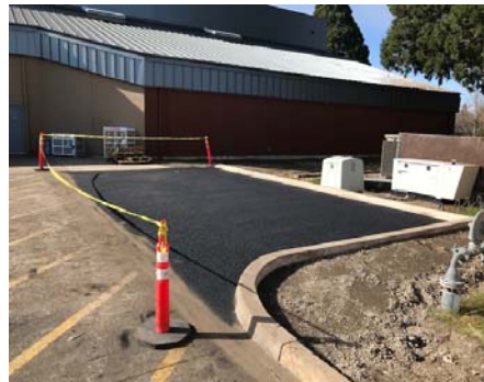
Equipment and new parking
